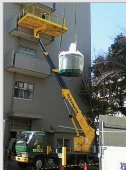
Cryogen-free 7T split pair for EPR with integrated variable temperature insert being installed in Kochi, Japan
